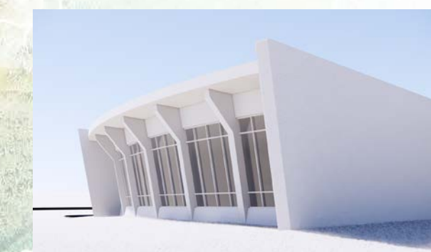
SOUTHERN FACADE. The columns are "branching" out to support overhang for shading.
